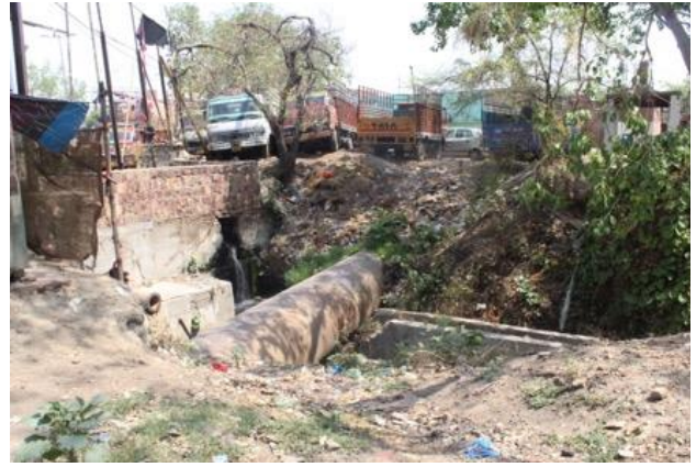
Figure 54Agra: Clogged drain
